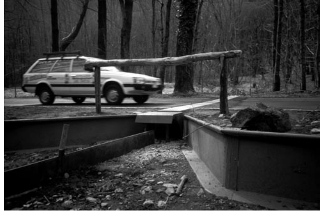
Fig. 1. Photograph of an underpass and barrier wall system near Arcegnò, Switzerland. The picture shows an entry to an open-top (ACO) tunnel and a metal barrier wall. The barrier wall has a zigzag shape. Note (i) the walking surface along the barrier wall and (ii) that the upper end of the barrier wall is ground level with the surface of the road. The wooden board helps to direct amphibians towards the tunnel entry. Photograph by Silvia Zumbach.
