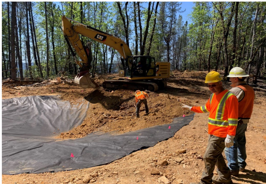
Figure 1. Pre-fire construction on wetland #11, spring, 2021.
